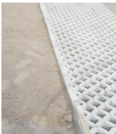
Gambar 7. Penyusunan material paving block grass block
