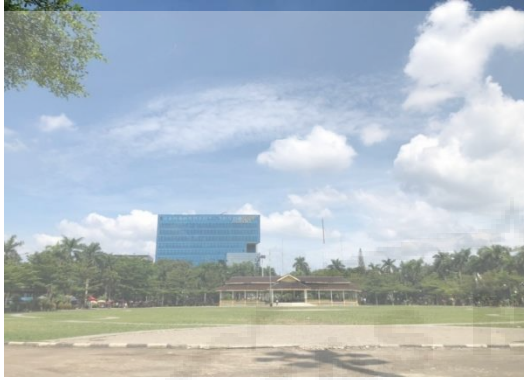
Fig: Merdeka Square Conditions, Source: Doc. Private June 26, 2021
