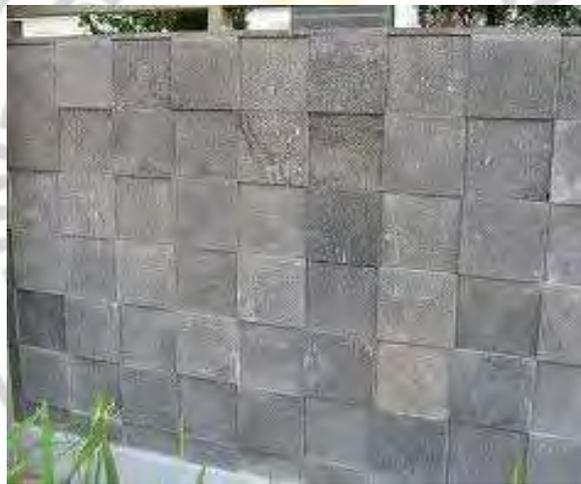
**Gambar 4.9. Tampak Depan Pasangan Dinding Dipasang Batu Alam**
