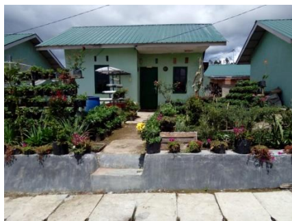
Figure 1. House of Siosar community relocation
